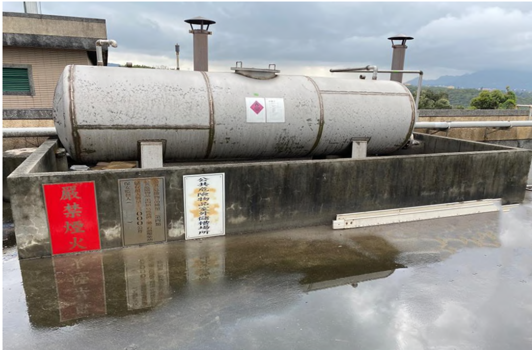
Above ground installation of diesel storage tanks with surface and associated pollution prevention facilities
