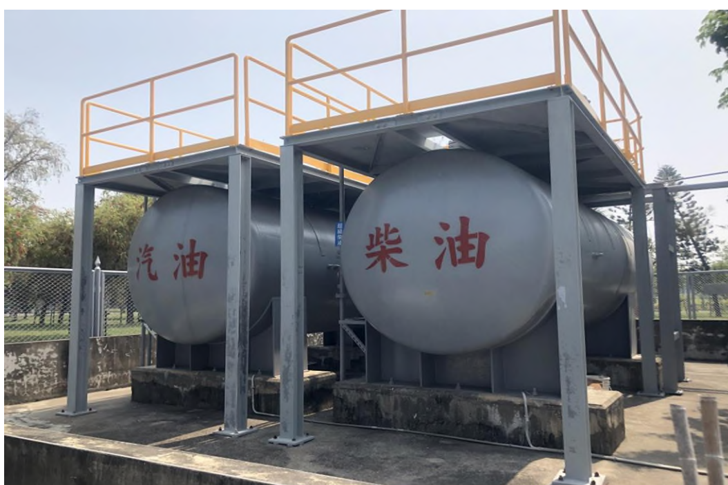
Above ground installation with gasoline and diesel storage tanks and associated pollution prevention facilities
