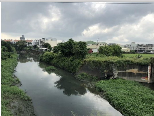
鹽行堤防 17 號水門 < 23°02'34.0"N 120°13'43.0"E >
