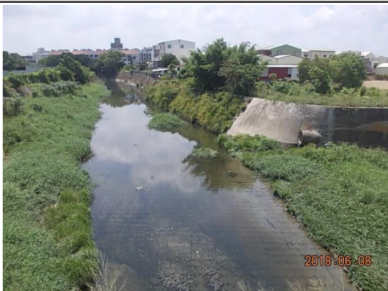
鹽行堤防 17 號水門 < 23°02'34.0"N 120°13'43.0"E >
