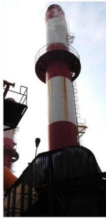
C. Power plant
